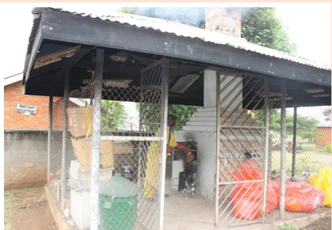
**Burning some of the waste at the repaired incinerator at Gulu Hospital**
